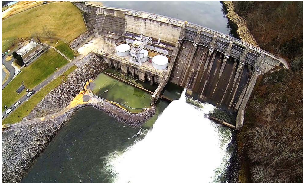
An aerial photo of Boone Dam, with Boone Lake behind it and its waters spilling into the South Fork Holston River. (Photo credit: https://tunnelingonline.com/nicholson-treviicos-jv-named-foundation-contractor-for-boone-dam-cutoff-wall/ )
